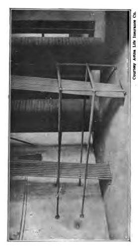
Pipe Railing Around Rope Drive where It Passes through Concrete Floor.
